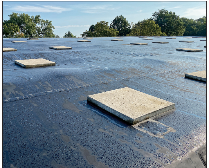
Delaminated Areas of Gym Roof
